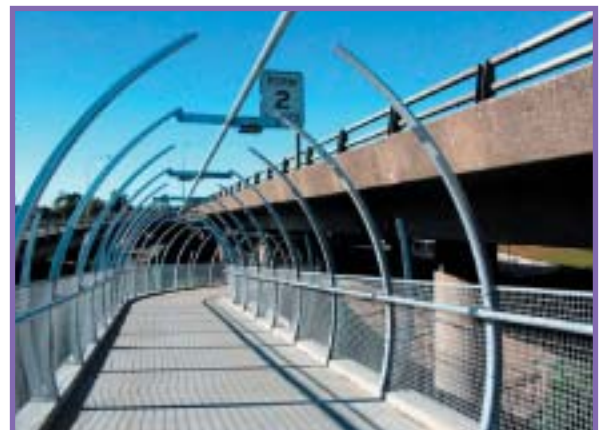
New cycling facility at Silverwater, completed in 2003
