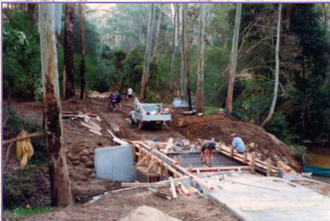
Brown's Waterhole Cycleway construction
