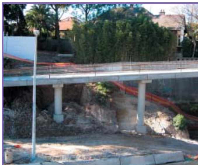
Exit Ramp at Merremburn Ave, Naremburn
