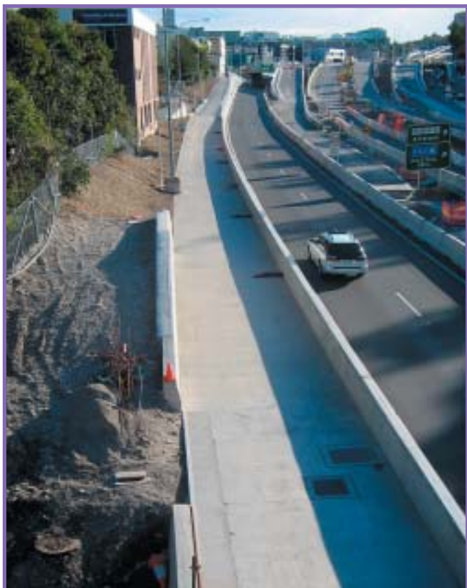
alongside Gore Hill Freeway looking west of Hampdon Rd, Artarmon
