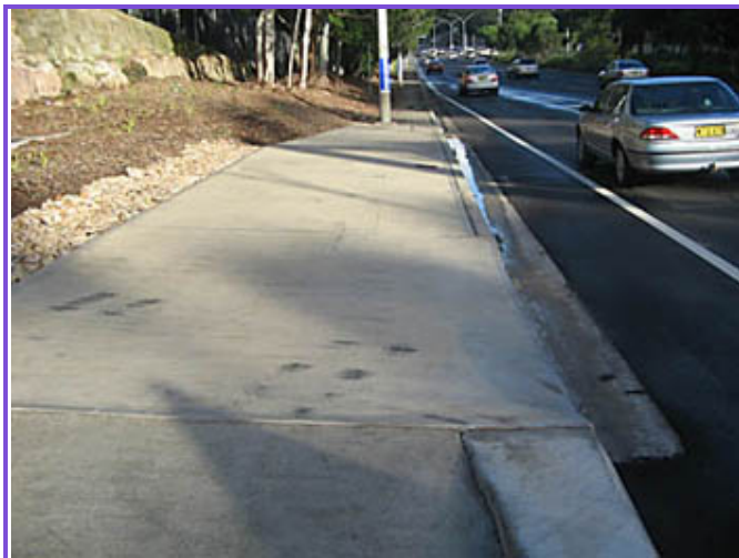
One option beyond the security gate is to join the motorway: the lane rapidly narrows and Brook St feeds in on the left
