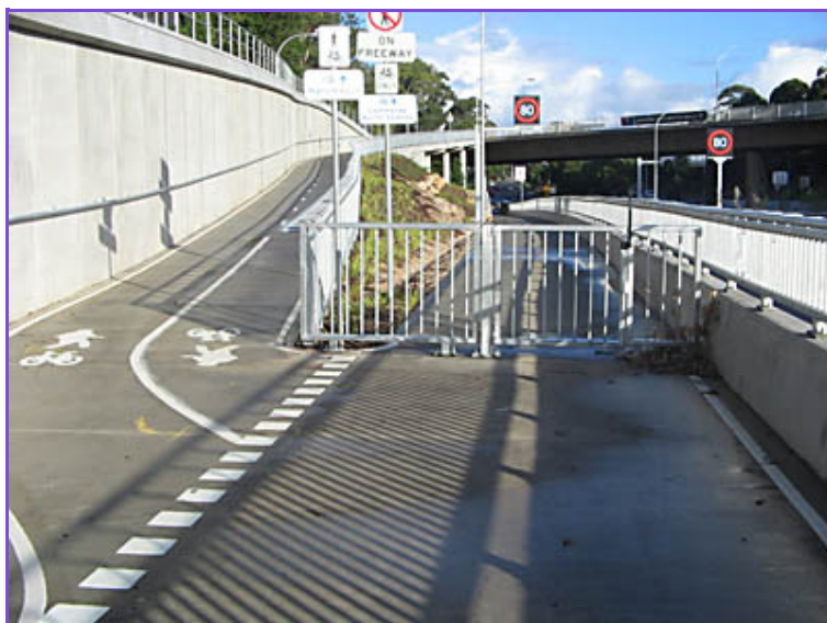
Gore Hill Freeway bike path, Naremburn. Merremburn Ave exit ramp OR through the secure fence to the motorway
