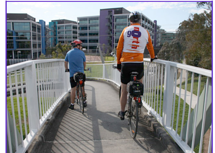
Checking connectivity to the overpass into Macquarie Park employment area
